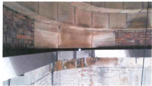
2.) Gutter behind stone work
