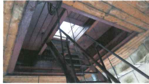
1.) Showing roof hatch and ladder B
