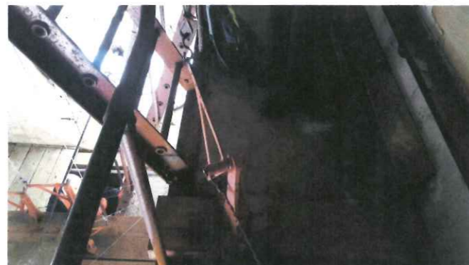
4.) Showing platform below hatch
